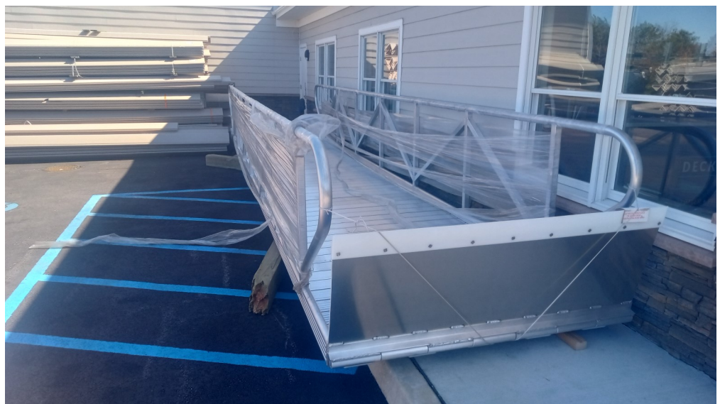
New Ramp for Dinghy Dock
